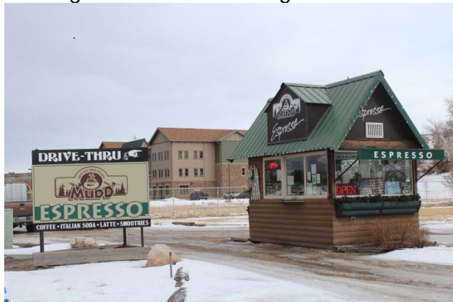
Existing coffee stand and sign:
